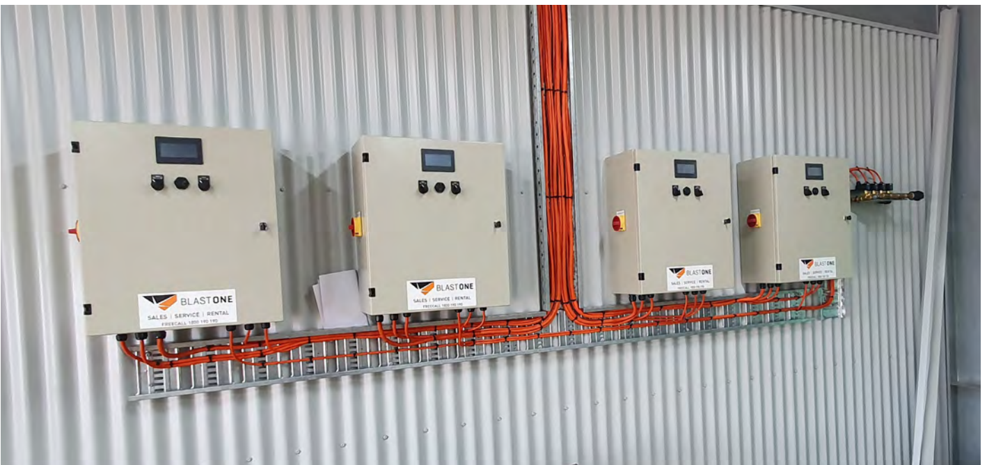
CONTROL CUBICLE FOR 8 FAN SYSTEM
