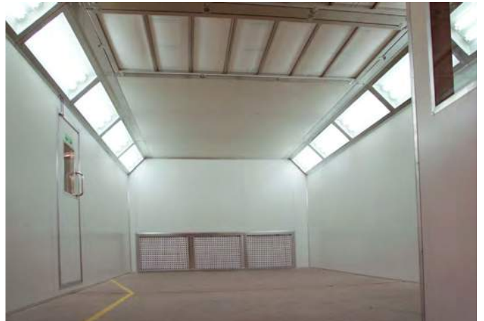
SEMI DOWN-DRAFT SPRAY BOOTH/CURING OVEN
